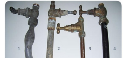
1. Lead, 2. Galvanized, 3. Copper, 4. Plastic
